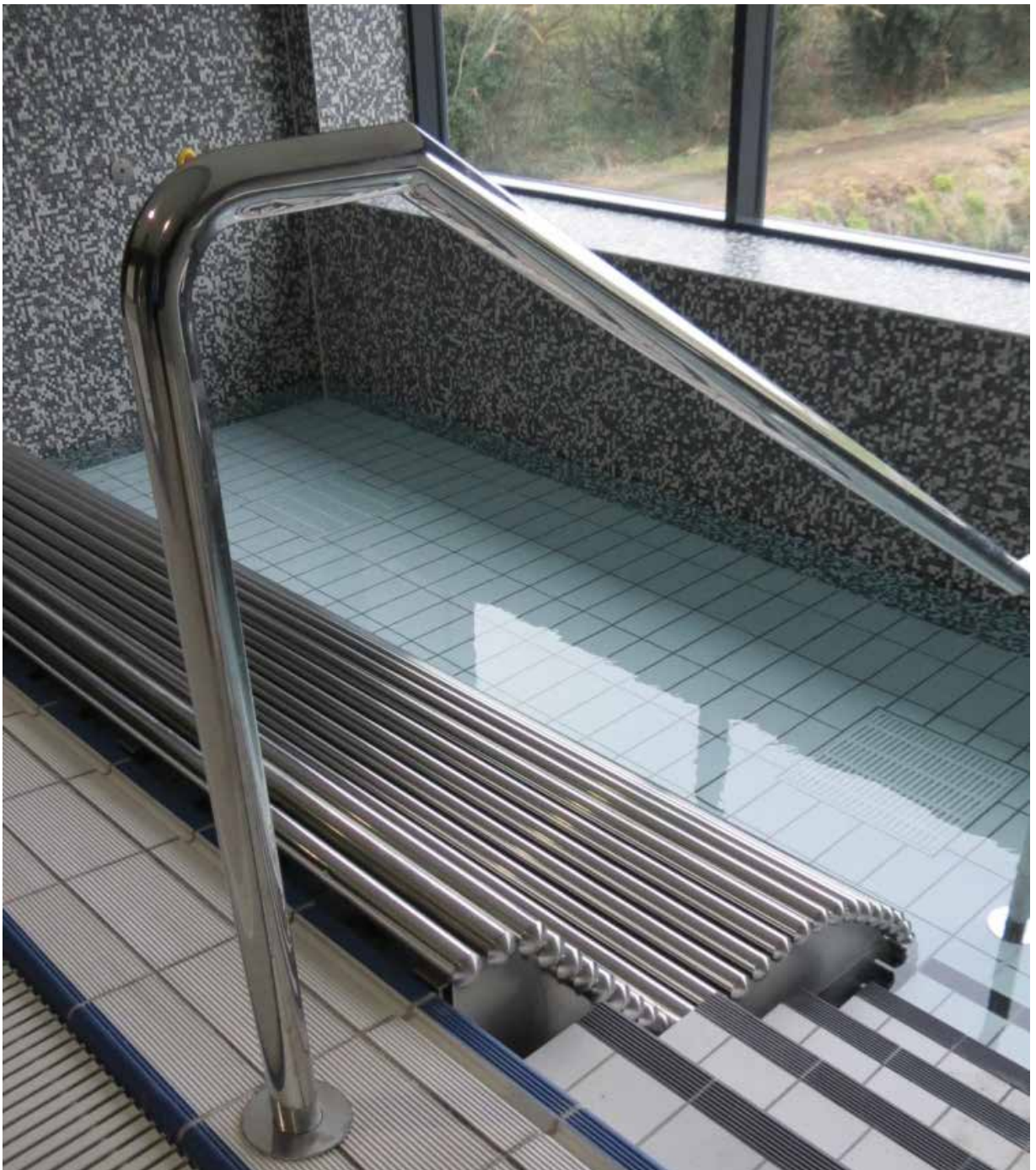
Contrasting step nosings and handrails to spa pool (Newry Leisure Centre)
