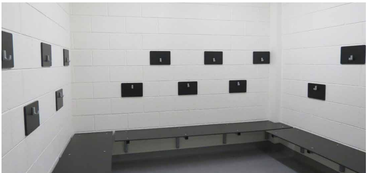
Alternate hooks fitted within inclusive team changing room (contrasting hooks and backboards) - Newry Leisure Centre
