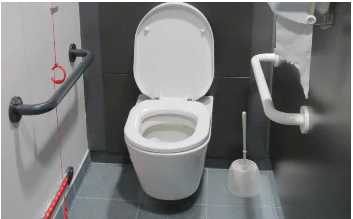
Ambulant accessible WC cubicle within inclusive toilet area (Foyle Arena, Derry-Londonderry)
