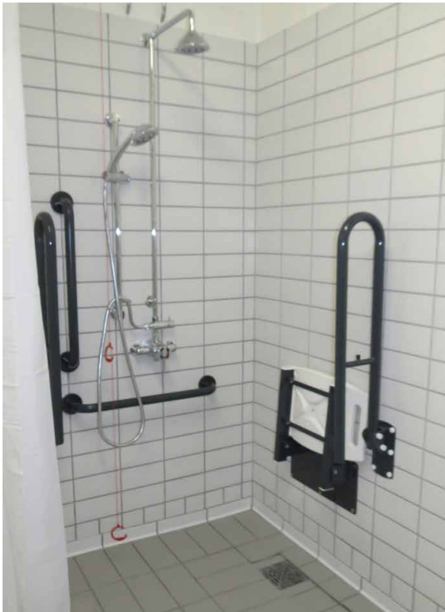
Wheelchair accessible incorporated shower provision within inclusive changing area (Newry Leisure Centre)
