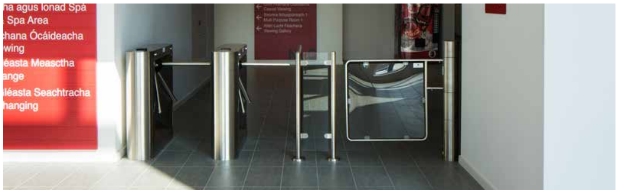
Accessible pass-through gate for inclusive access in reception, Newry Leisure Centre - (image courtesy of Donal McCann Photography)
