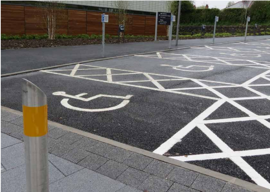
Accessible Parking Bays (Foyle Arena, Derry-Londonderry)
