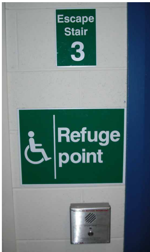
Refuge clearly signed (The Torrent Complex, Donaghmore)
