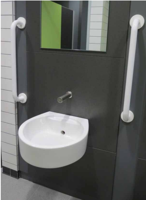
Lowered wash hand basin and urinal provision, including contrasting grabrails, within inclusive toilet areas (Foyle Arena, Derry-Londonderry)
