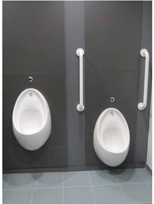
Lowered wash hand basin and urinal provision, including contrasting grabrails, within inclusive toilet areas (Foyle Arena, Derry-Londonderry)
