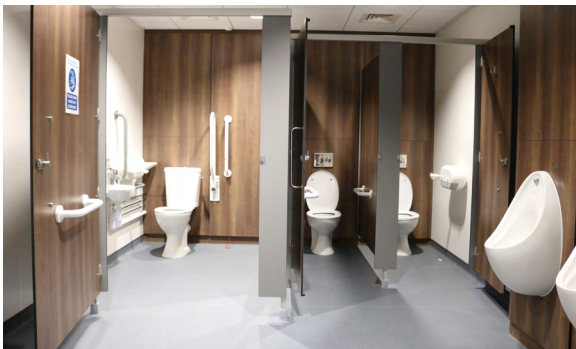
Image 4 - Wheelchair accessible WC cubicle and ambulant accessible WC cubicle incorporated within an inclusive toilet block
